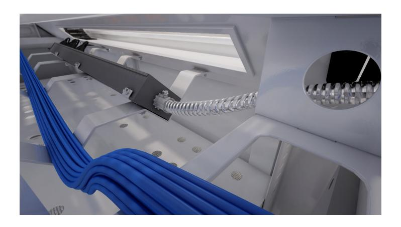
Power and data cabling is routed, separated and protected inside the desk raceway to maximize space and clearance for technology.
